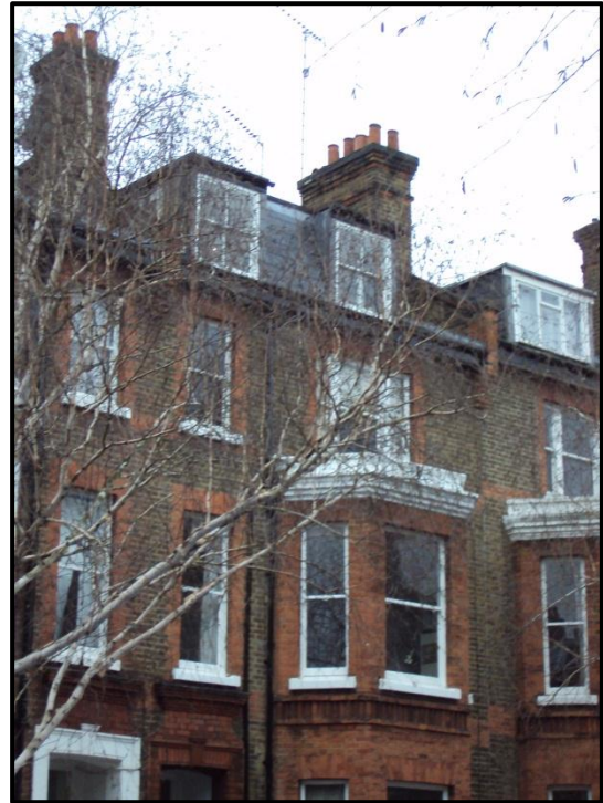
Fig. 1- Existing view: Front elevation showing flat roofed dormers in situation
